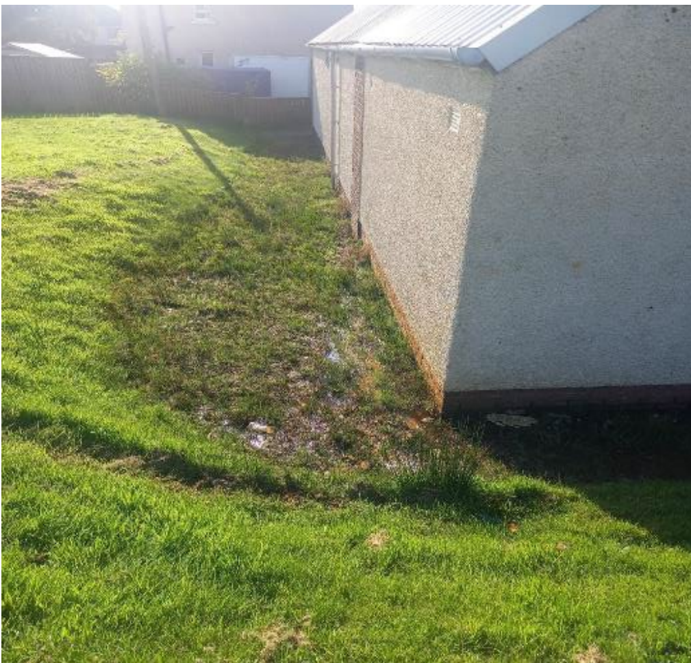
E) Loch Park Image – Front / Side View (Rough Casting / Missing Gutters & Vandalism)
